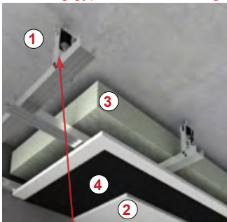
Typical application of sound insulating gypsum board ceilings
